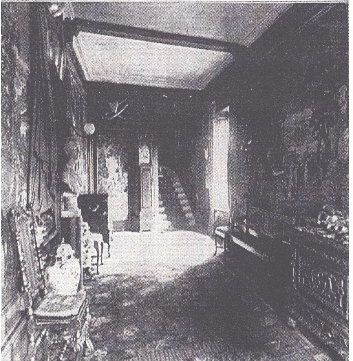
The corridor, looking east
